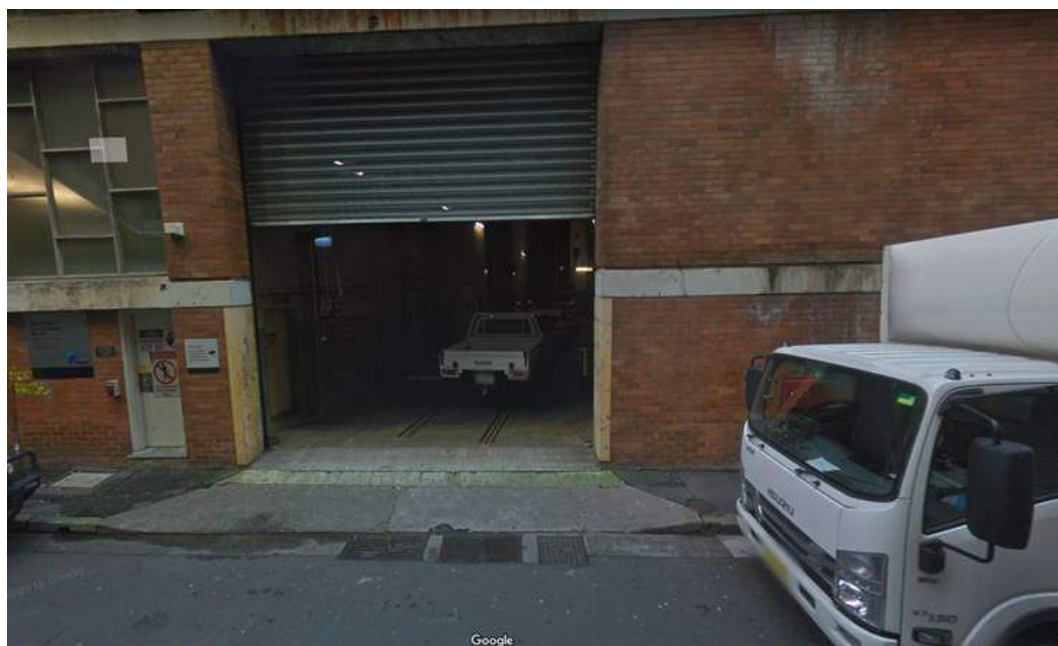
Figure 19 - Existing Ausgrid vehicular entry
